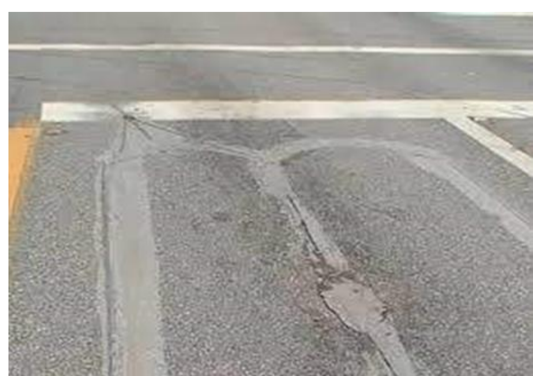
Figure 1: Inductive Loop Detector Embedded in the Road Pavement used in PTC Program
