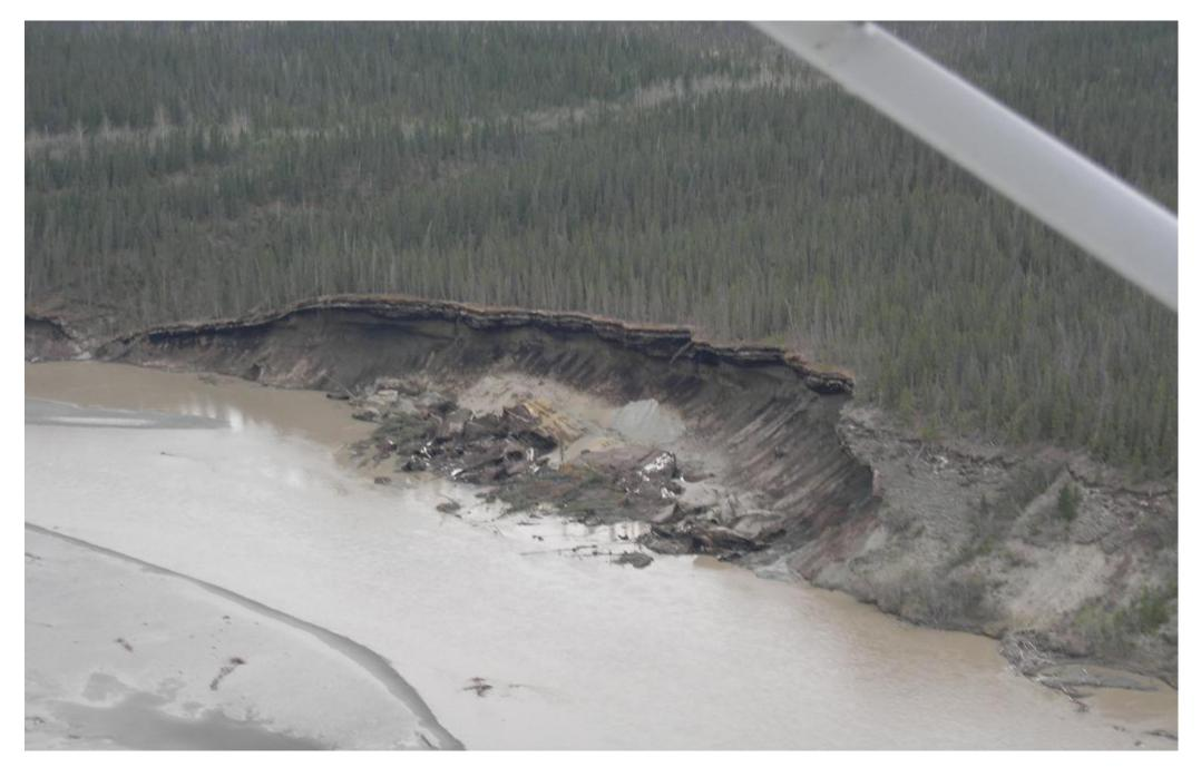
Figure 2. Slope failure due to drawdown. (photo by Neil F. Humphrey)
