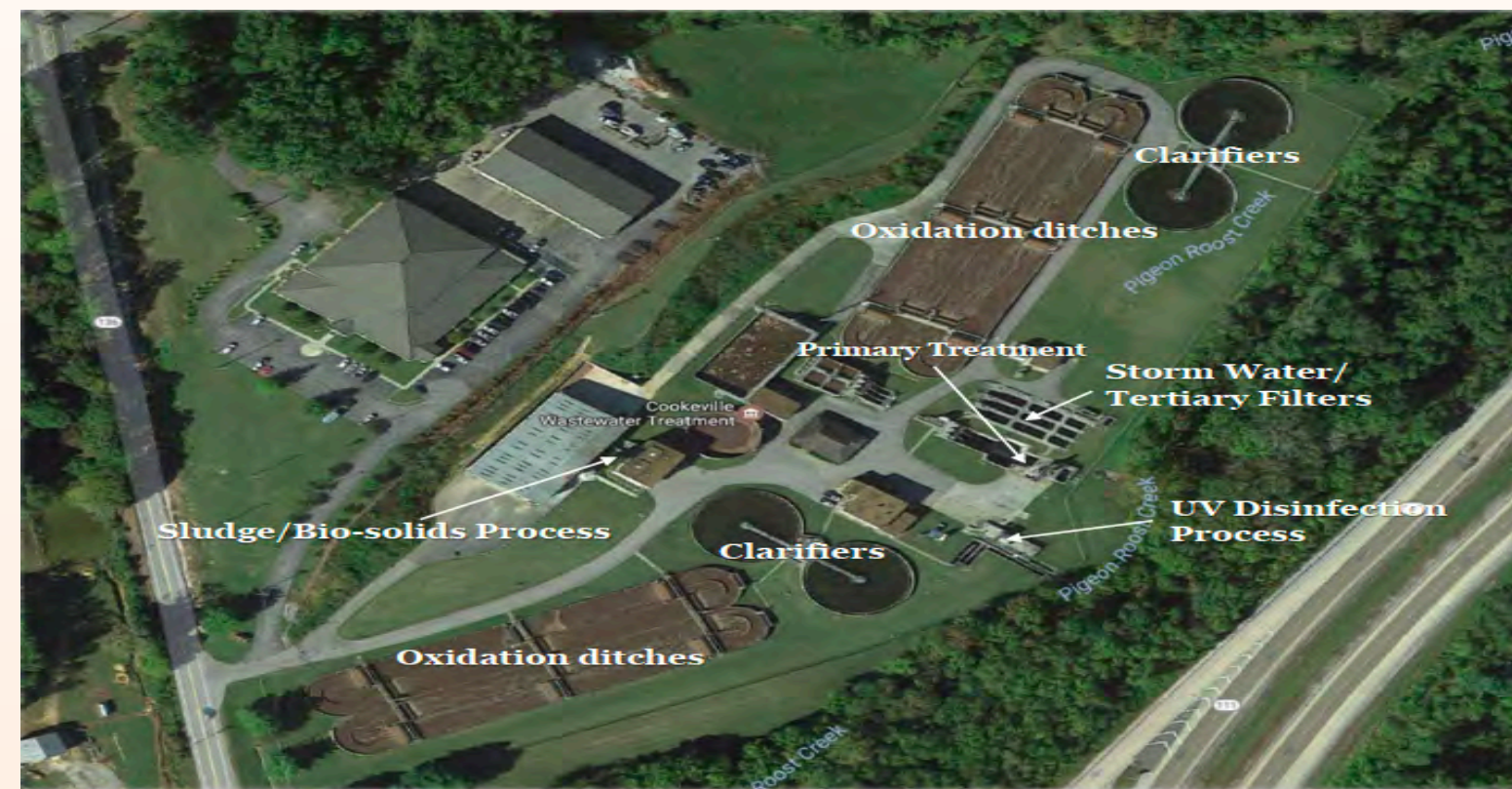
Fig. 1 Cookeville Waste Water treatment plant Ref.Cookeville-tn.gov
