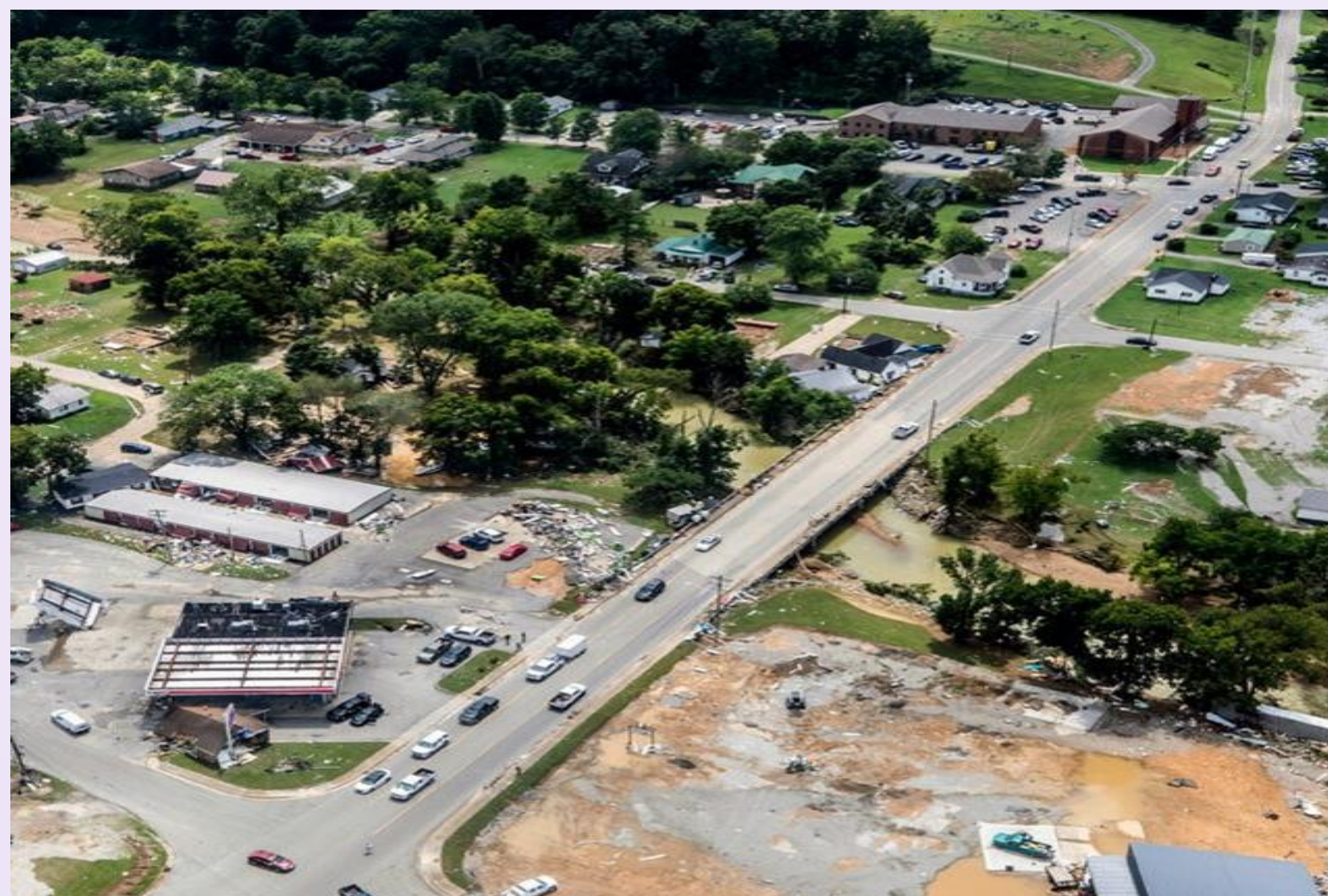
Figure 2. August 2021 flood damage in Waverly, TN (Source: The New York Times , 2021)
